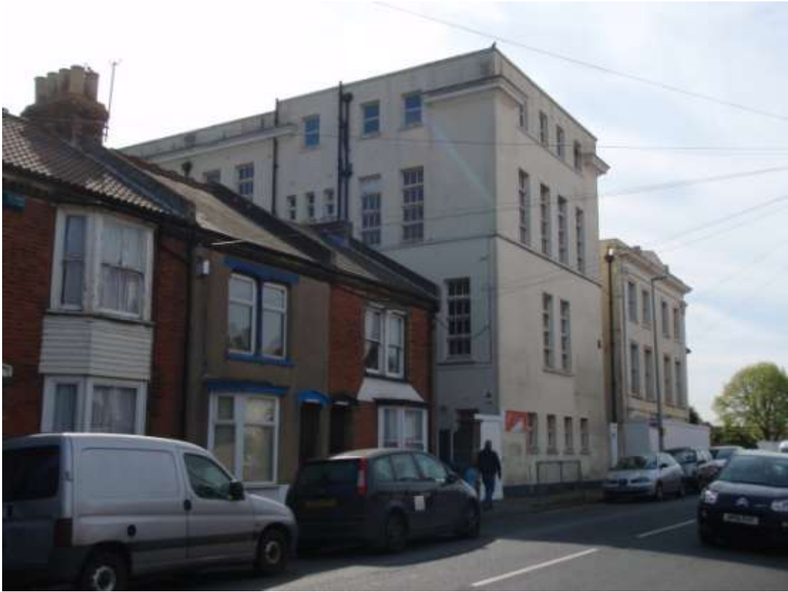
Plate 5. Front facade to Avenue Road of east extension (3)
