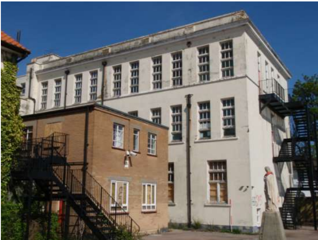
Plate 6. Rear view of east extension (3)
