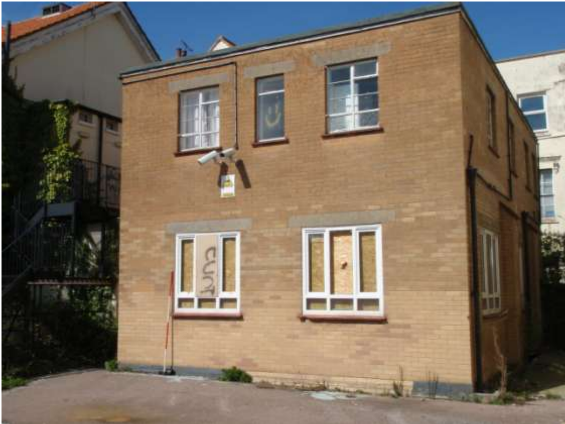
Plate 9. View of facade of Brick Infill Building (4) looking NNW
