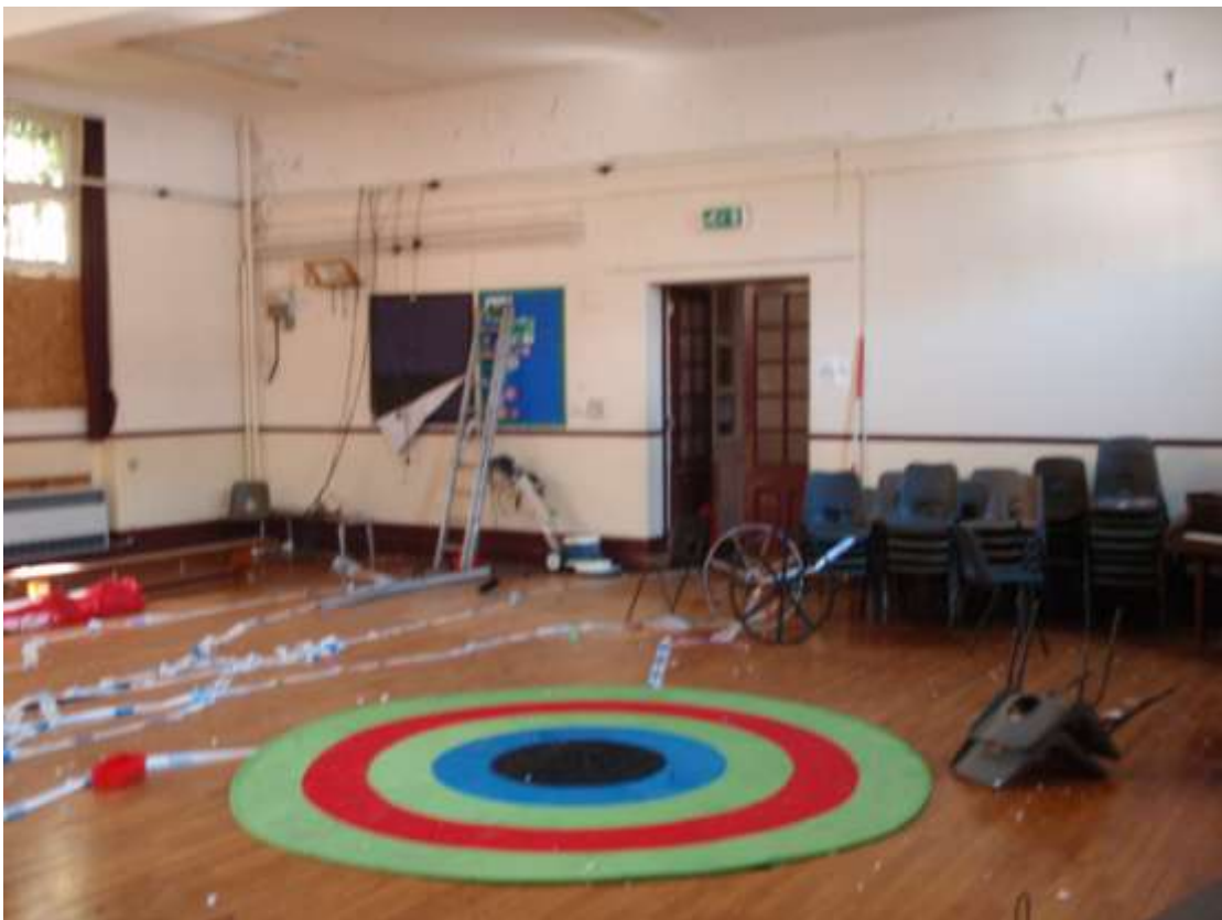
Plate 23. Ground floor assembly room East Extension (3)
