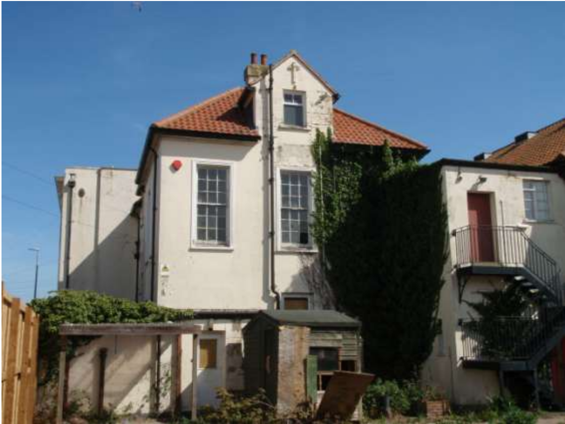
Plate 14. View of the West Extension (2) looking SSE
