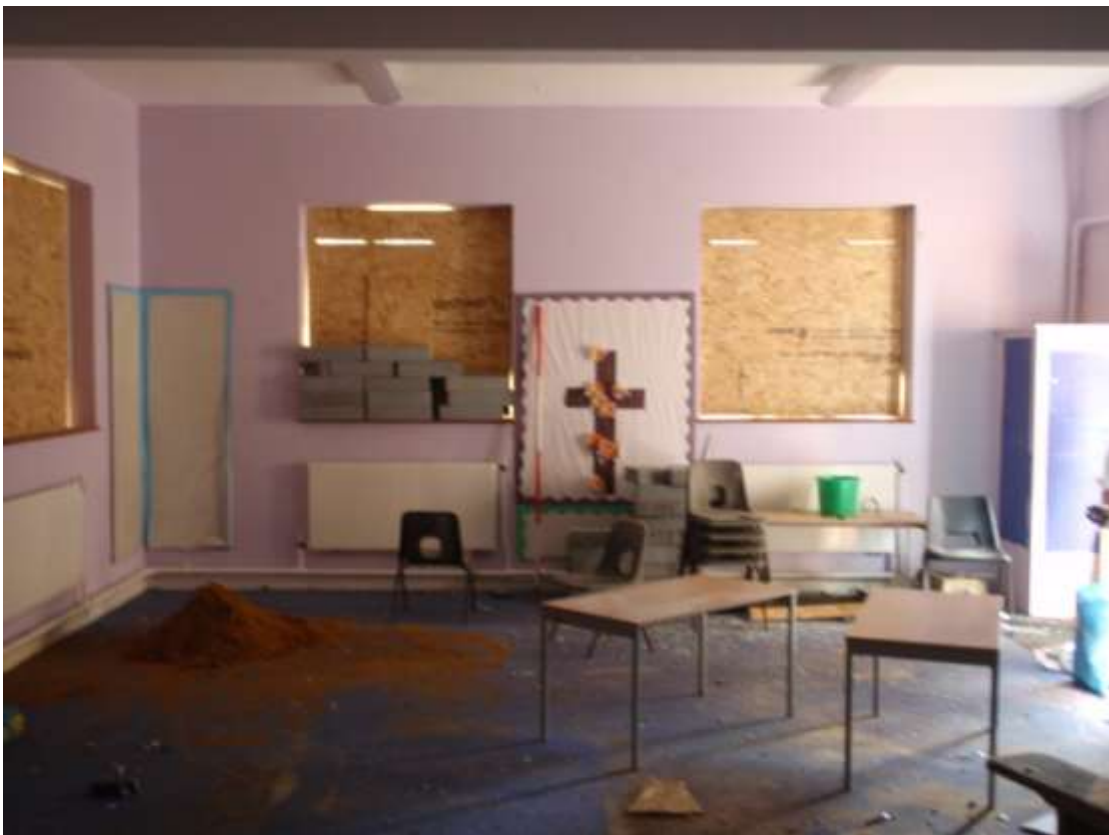
Plate 19. Classroom West Extension (2)
