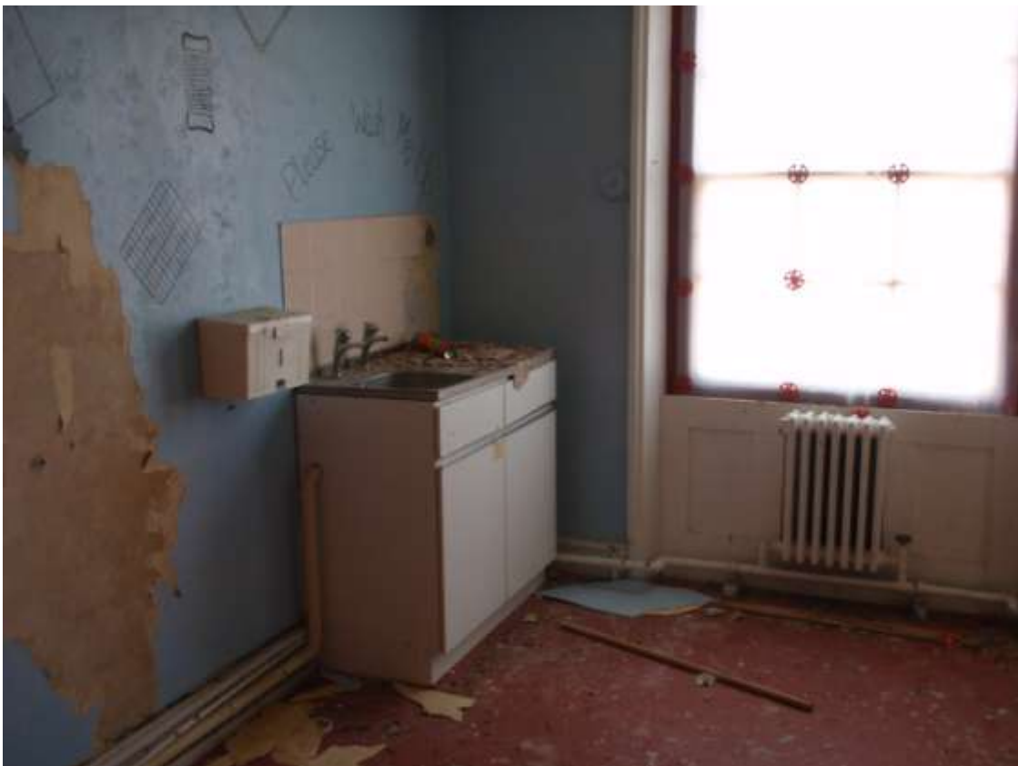
Plate 25. Ground floor kitchen East Extension (3)
