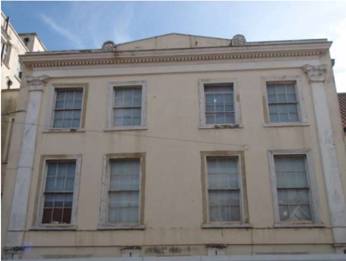
Plate 1. Listed building: front elevation to Avenue Road
