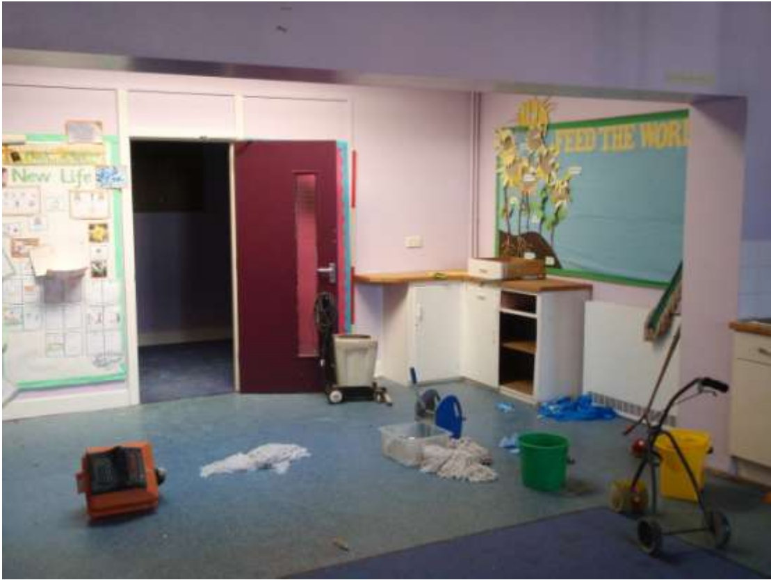
Plate 18. Classroom West Extension (2)
