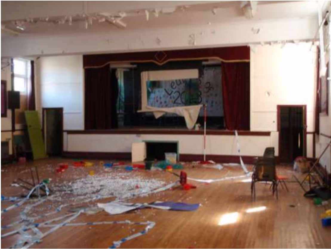
Plate 22. Ground floor assembly room East Extension (3)
