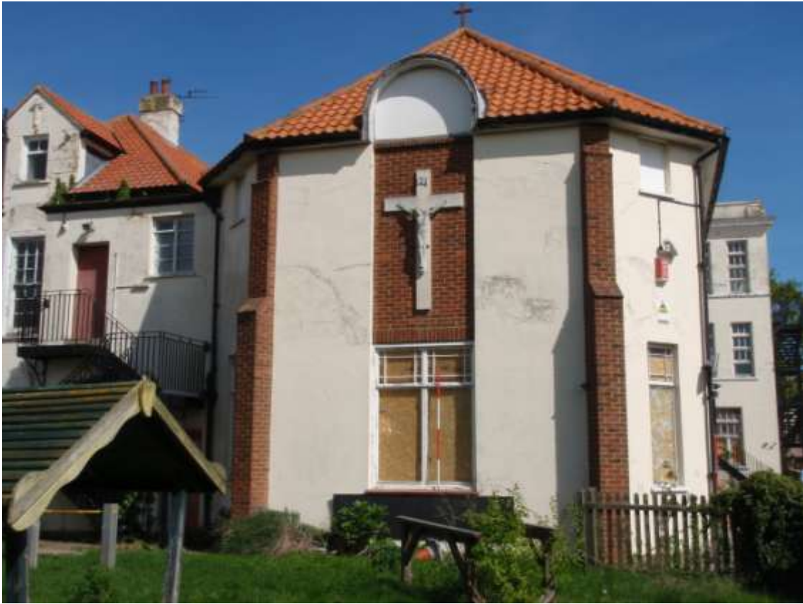
Plate 12. View of the Chapel (1) looking E
