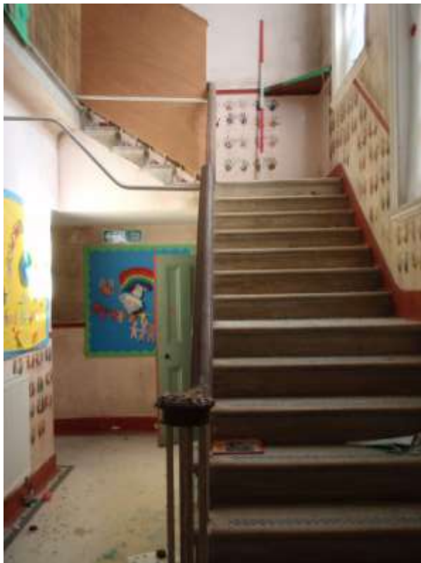
Plate 21. Staircase East Extension (3)
