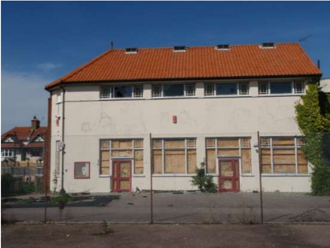
Plate 10. Facade of the Chapel (1) looking N
