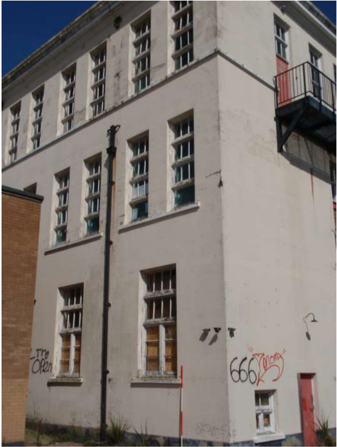
Plate 7. Detailing of east extension
